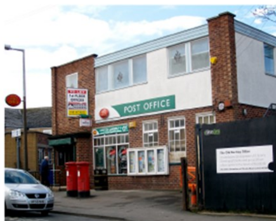
Post Office, Maple Road
